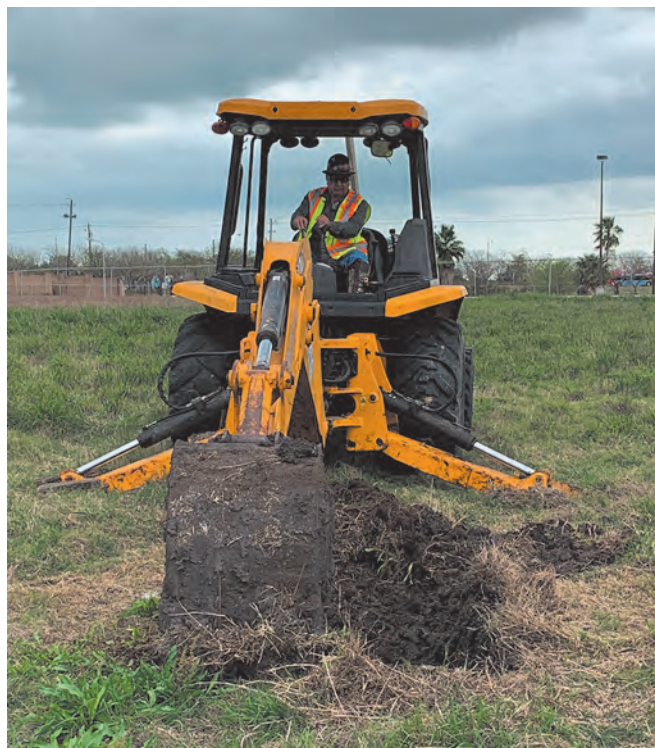
Figure 5. A backhoe was used to excavate holes for GTS target placement.
