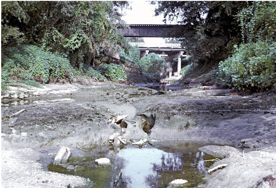
Figure 3. The Moodys Branch formation exposed at Town Creek in Jackson, Mississippi, (MGS locality 1) before the construction of a sewer line across the site. A railroad bridge and the South State Street bridge appear in the background. Picture (Kodachrome slide 155-5) taken in September of 1970.
