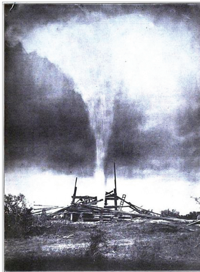
Figure 3. The Guffey No. 2 gasser ( Fuel Oil Journal 1916a, p. 115). Caption states an estimated flow rate of 100-125 MMCFGD.
